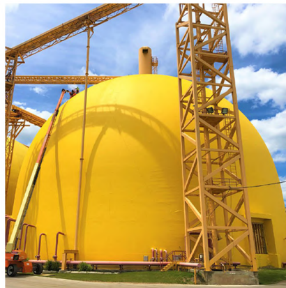
Cement Domes, Riverside, CA
