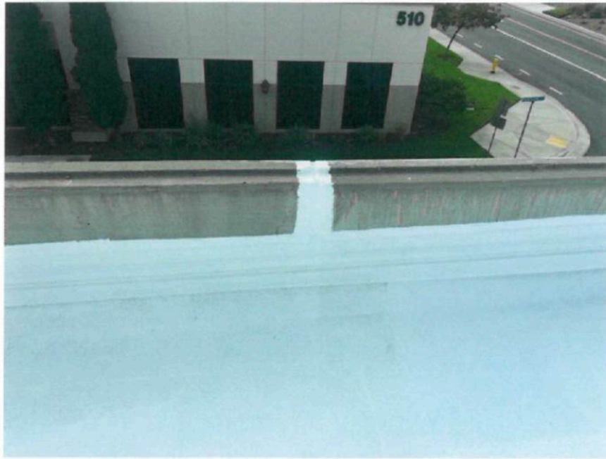
Completed Silicone roof system.
