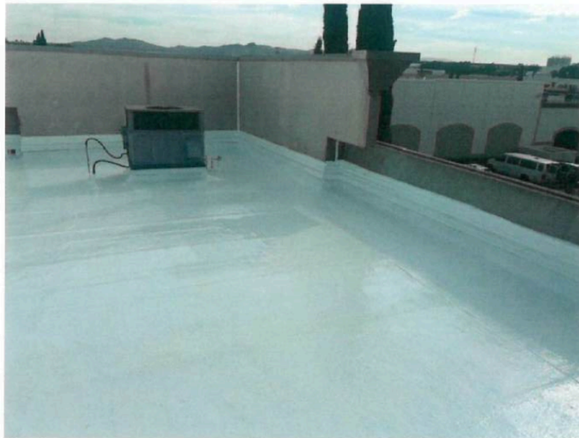
Completed Silicone roof system.
