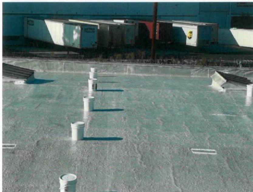
Gridding out the Silicone buckets for coating.
